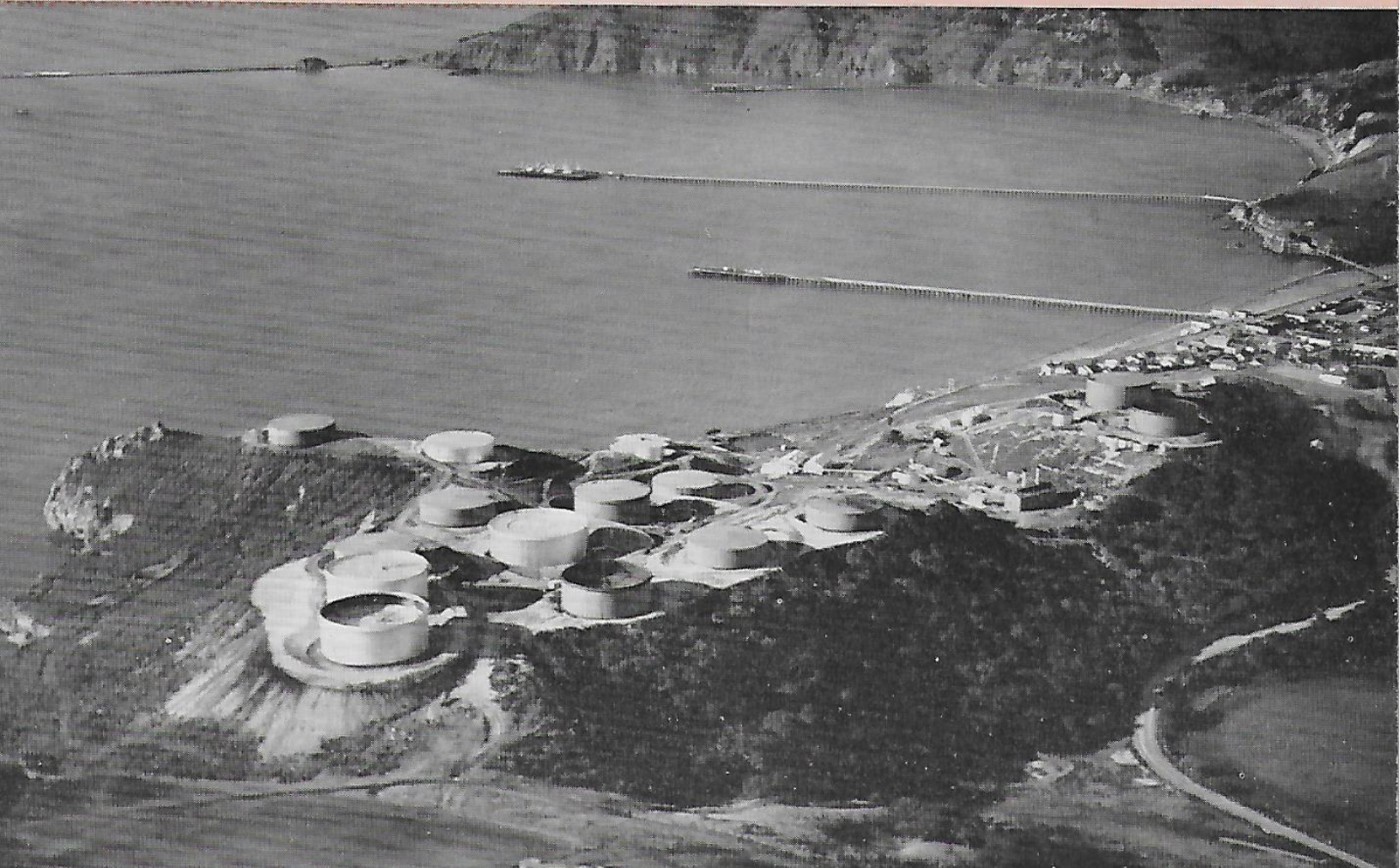
AVILA PUMP STATION OVERLOOKING PORT SAN LUIS, CALIFORNIA
