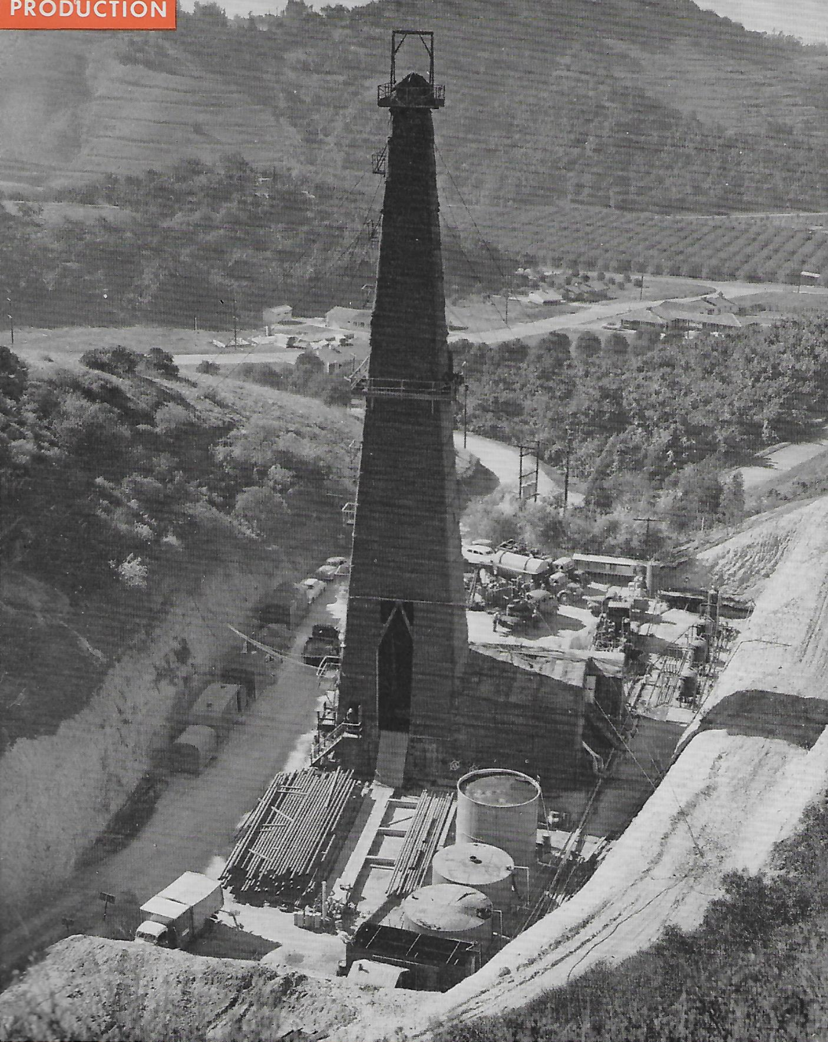
DRILLING OPERATIONS NEAR WHITTIER, CALIFORNIA
