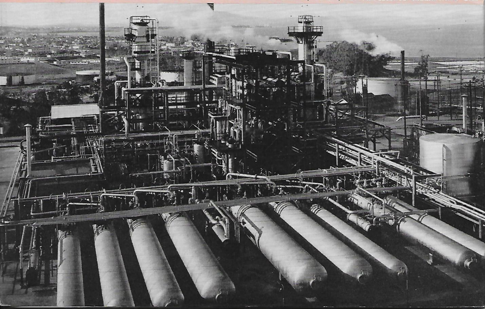
DUO-SOL UNIT, OLEUM, FOR PROCESSING LUBRICATING OILS
